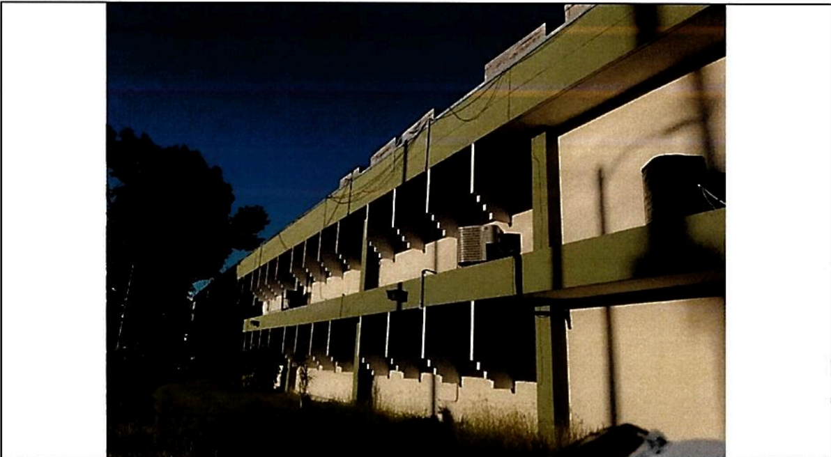
General View – Main Bldg. (Middle and High School)
